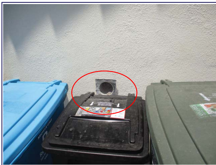
Improperly terminated clothes dryer exhaust duct.
