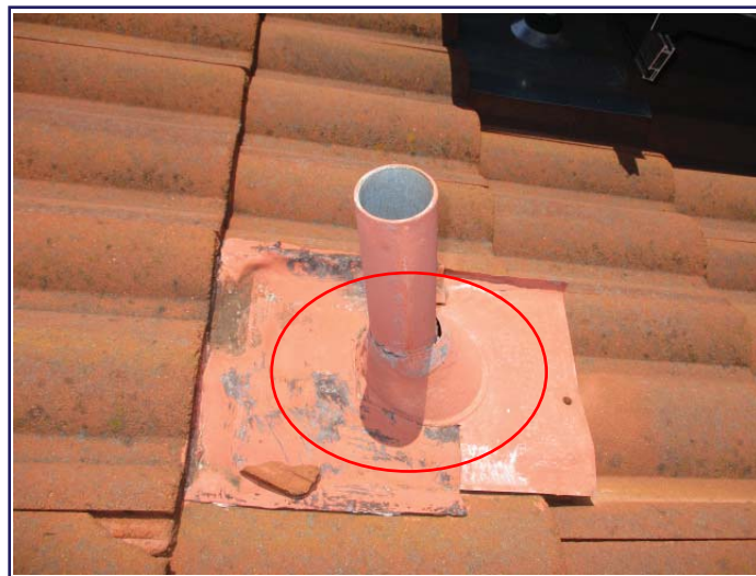
Unsealed plumbing vent flashings.
