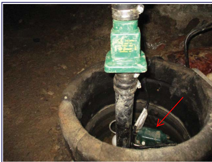
One of the sump pumps in the sub area.
