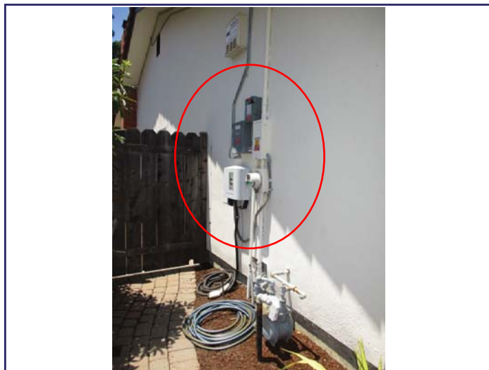
Main electrical panel and PV system equipment at the left front corner of the garage.
