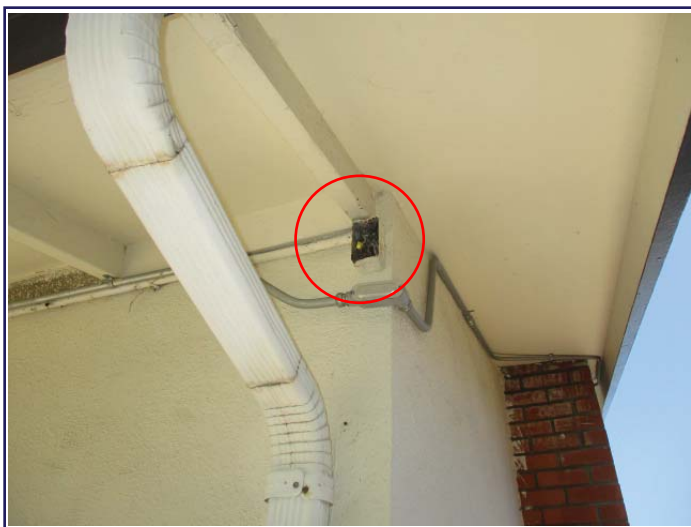
Uncovered exterior electrical junction box.
