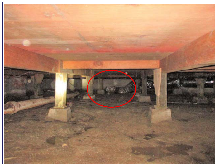
Disconnected duct and puddling water beneath the living room.
