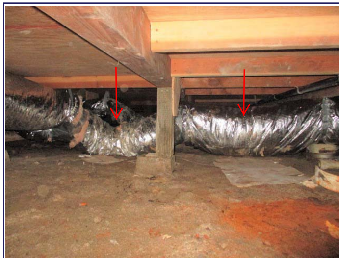
Ducting on the wet ground in the sub area.
