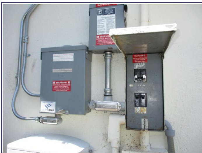
Main electrical panel and PV system panels.
