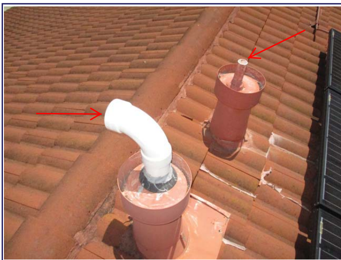
Improperly terminated furnace and water heater vents.
