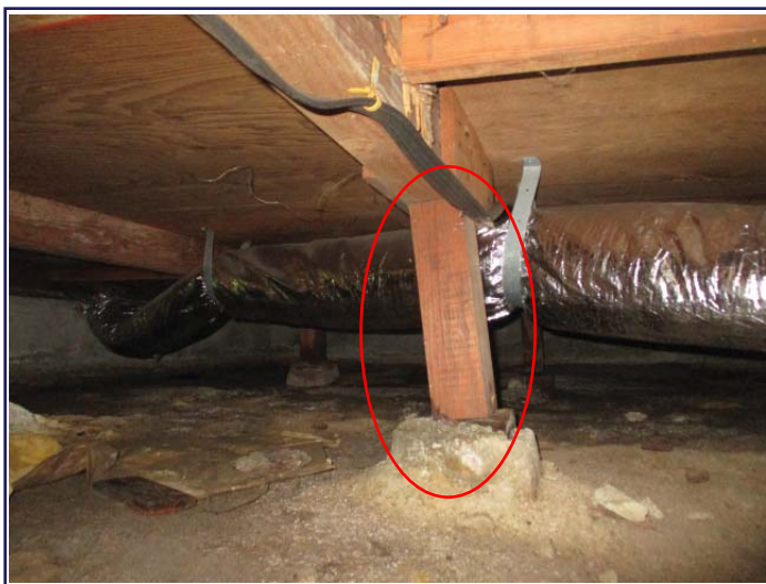
One of the out of plumb posts in the sub area.
