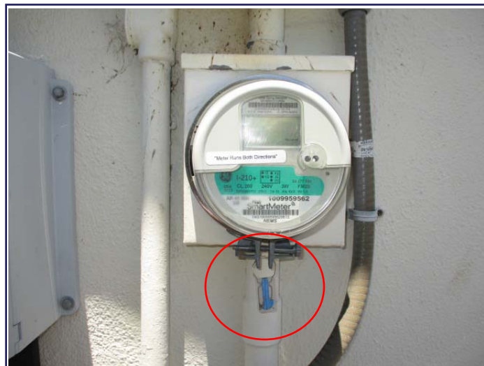
The electric supplier utility seal at the power meter was broken.
