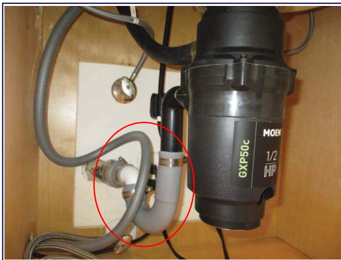
Improperly installed drain plumbing under the kitchen sink.
