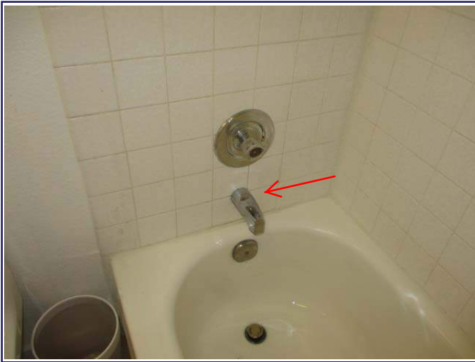
Unsealed tub spout flange.
