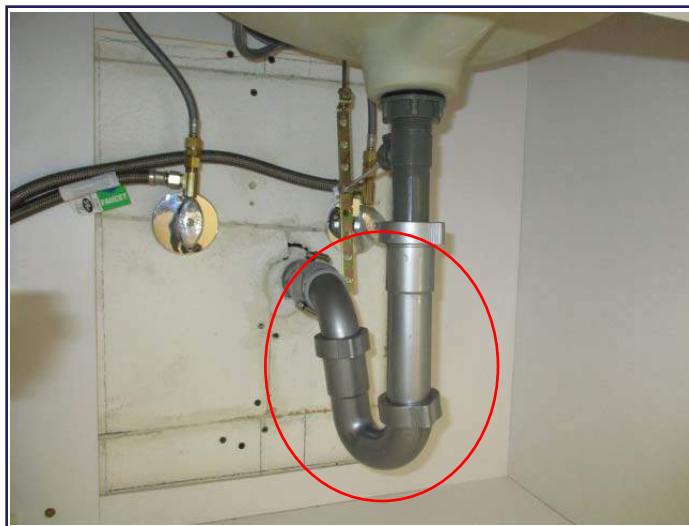
Improperly installed drain plumbing under the right bathroom sink.
