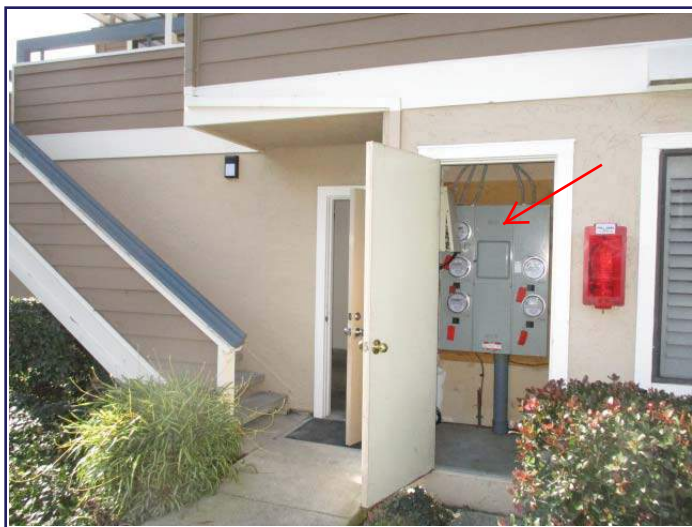
Main electrical panel in the exterior closet to the right of the exterior stairs.
