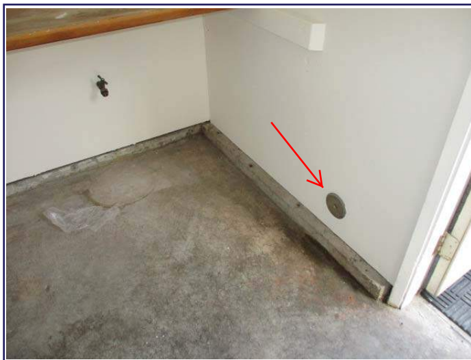
Main sewer clean out in the garage.
