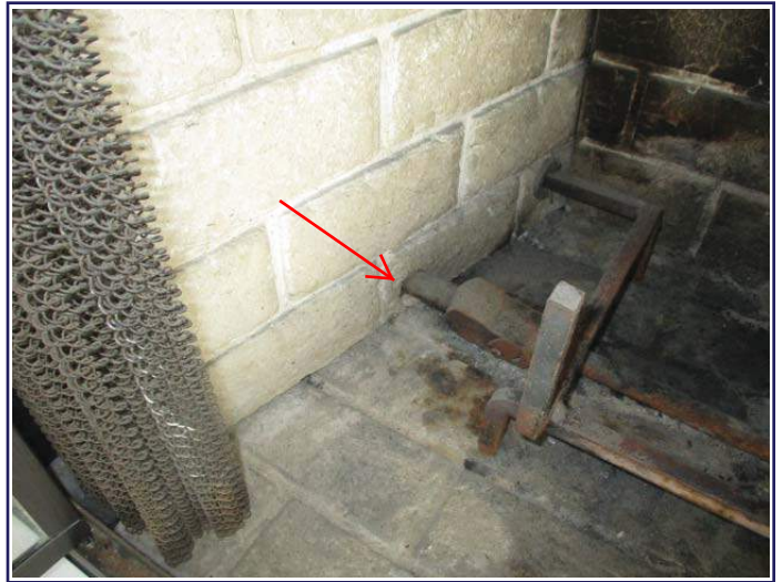
The penetration for the gas log lighter pipe in the fireplace was unsealed.
